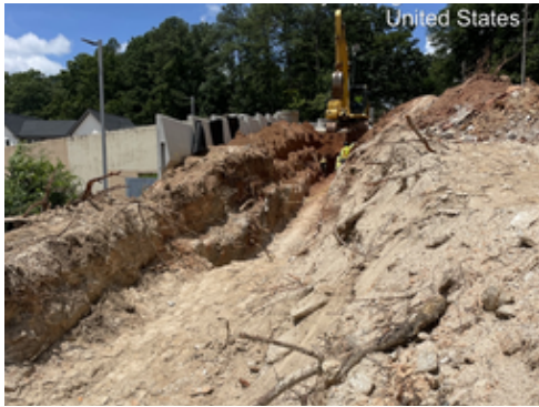
TS108 Stormwater Installation
