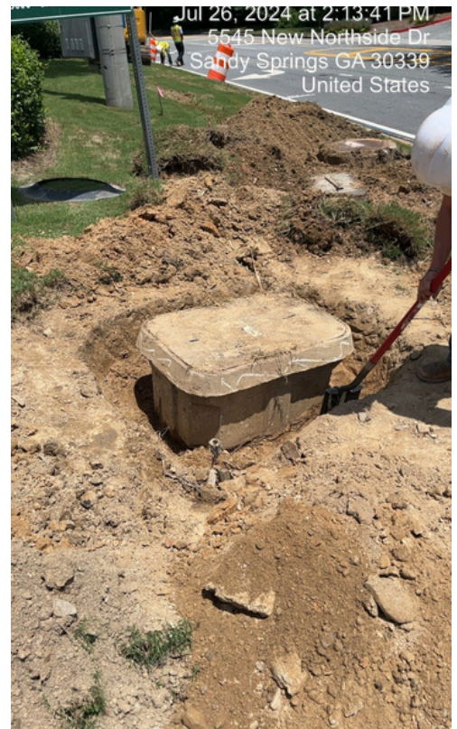
TS191 Curb and Gutter Installation
