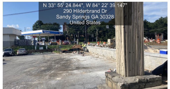
TS191 Wall construction
