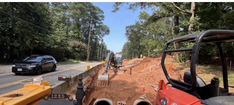
TS111 Stormwater Installation
