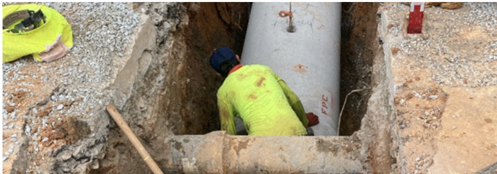
TS191 Stormwater Installation
