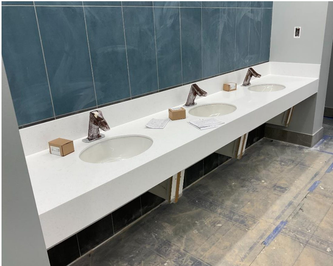
Restroom Countertops & Sinks at 3 rd Floor
