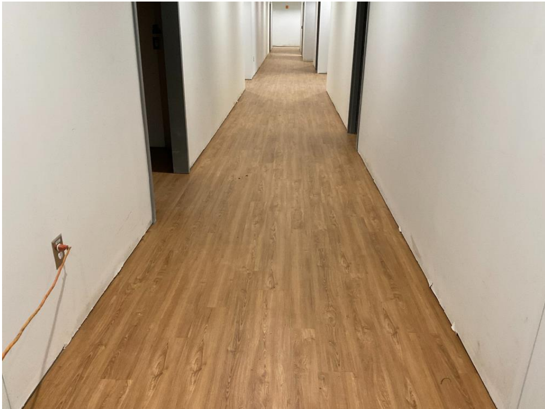
LVP at 2 nd Floor Hallway
