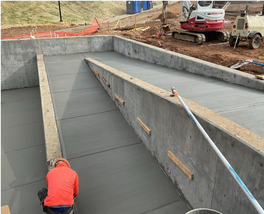
Freshly Poured Wall B Ramps
