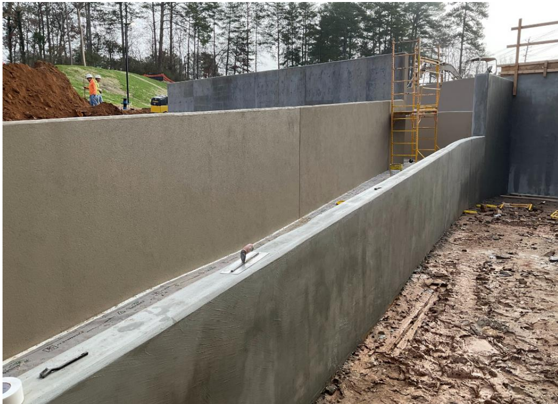
Stucco at Wall B Ramps
