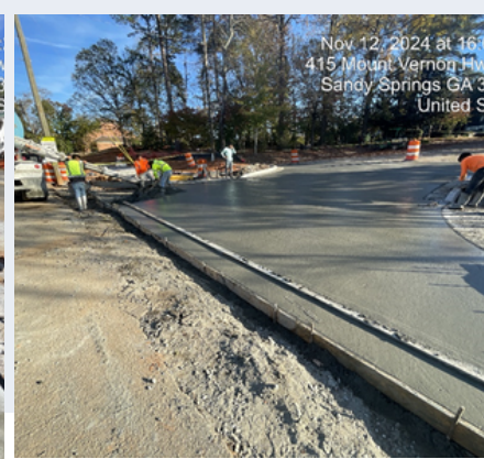
TS191 Multi-use path construction and Driveway Installation
