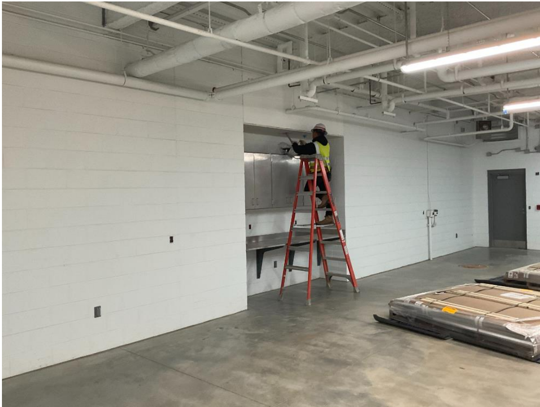
Sealed Concrete & Stainless Steel Countertops at Sallyport
