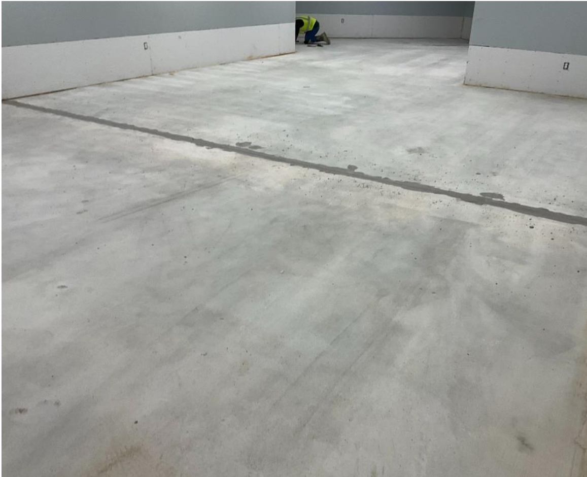
Flooring Prep Work
