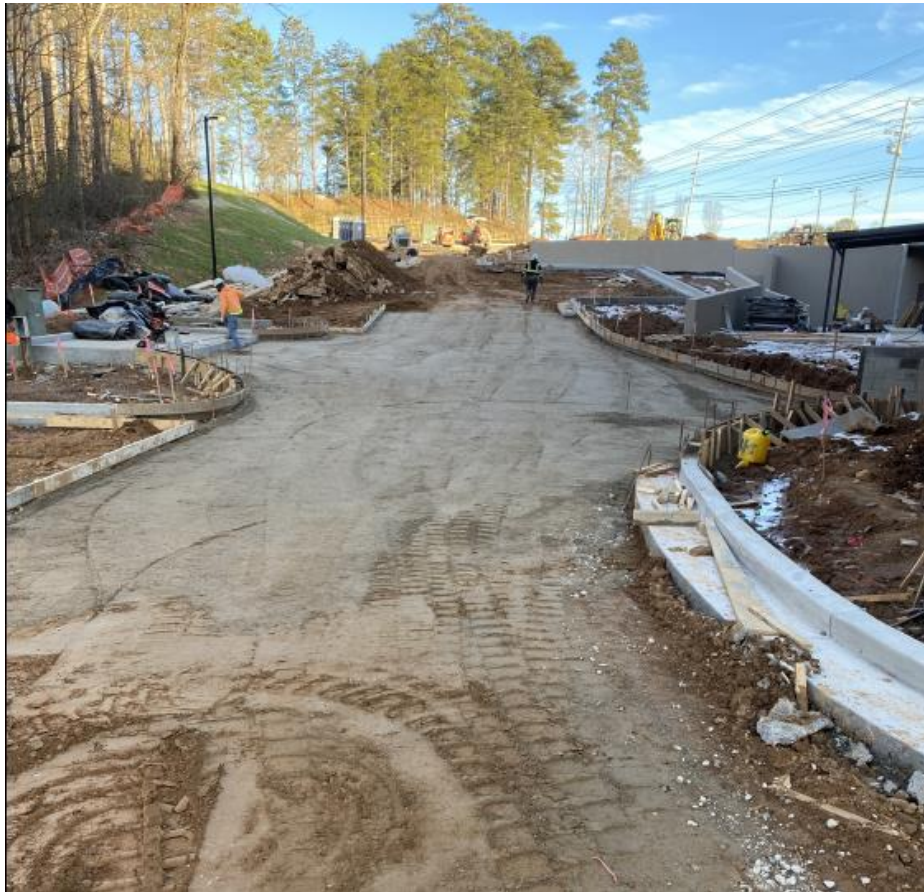
Prepping for Heavy Duty Concrete
