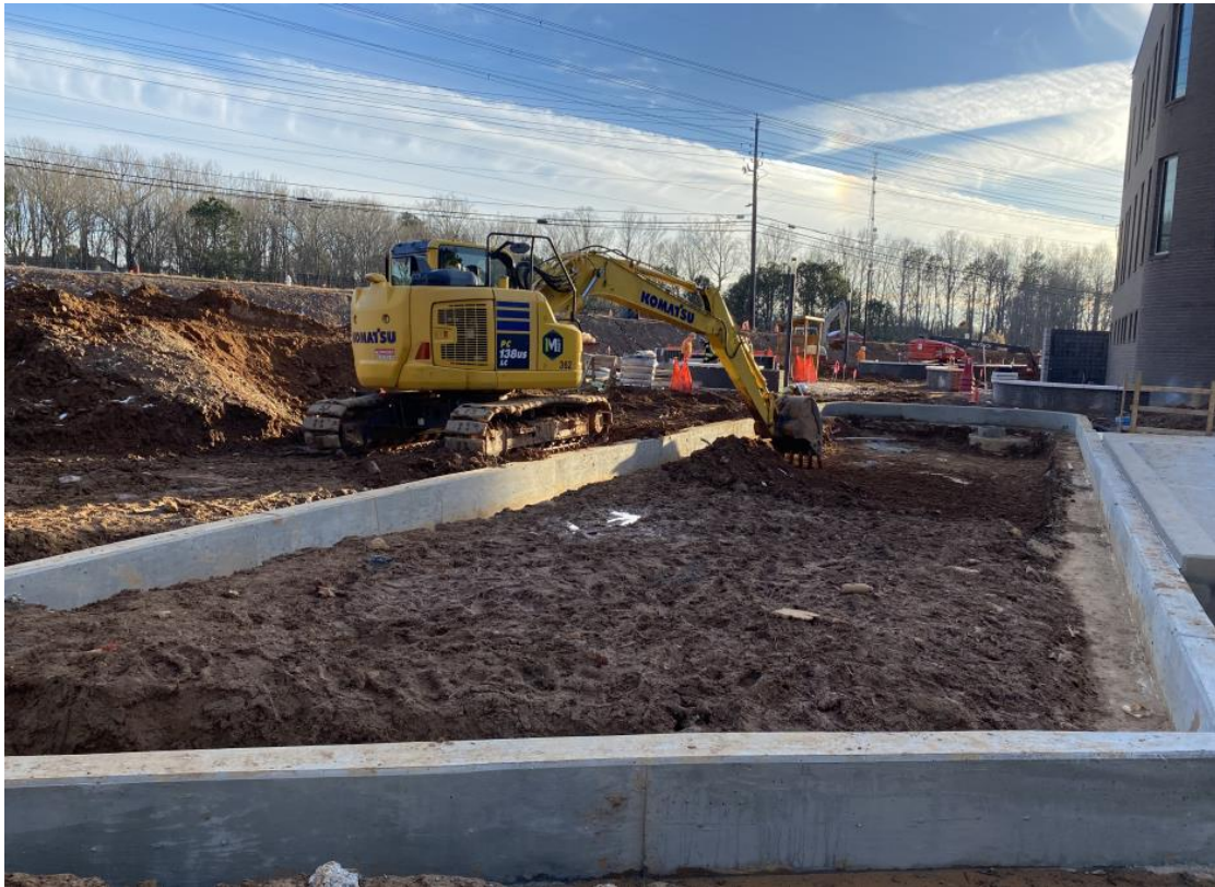
Excavating at Bio Cell
