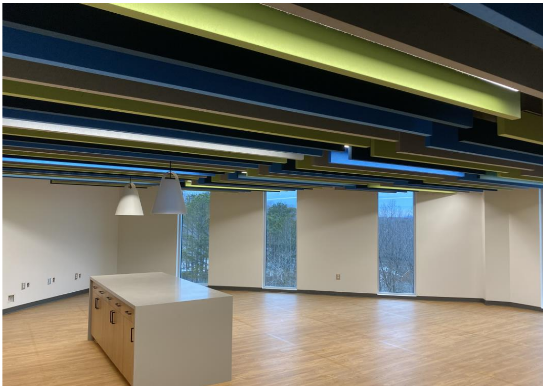
Ceiling Baffles at Breakroom
