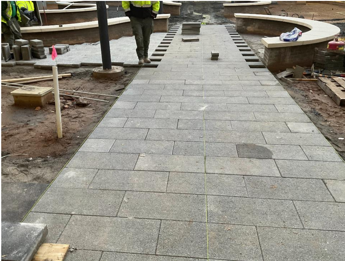
Pavers at Courtyard
