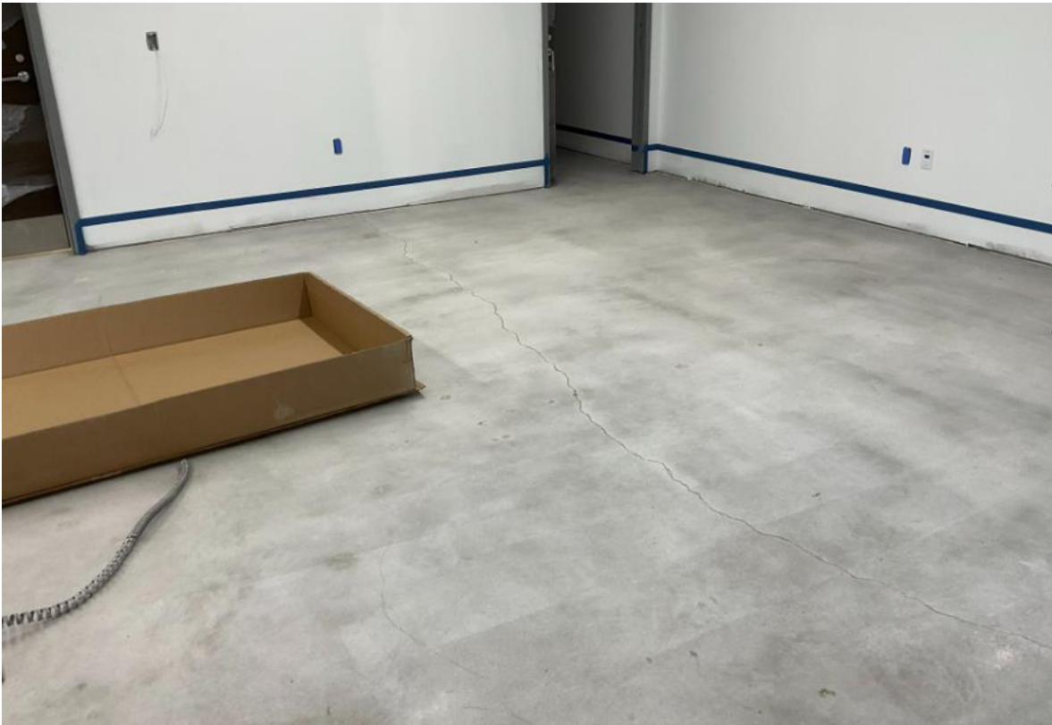
Prep for Epoxy Floor at Evidence Lab
