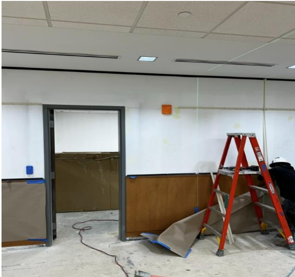
Millwork at Courtroom
