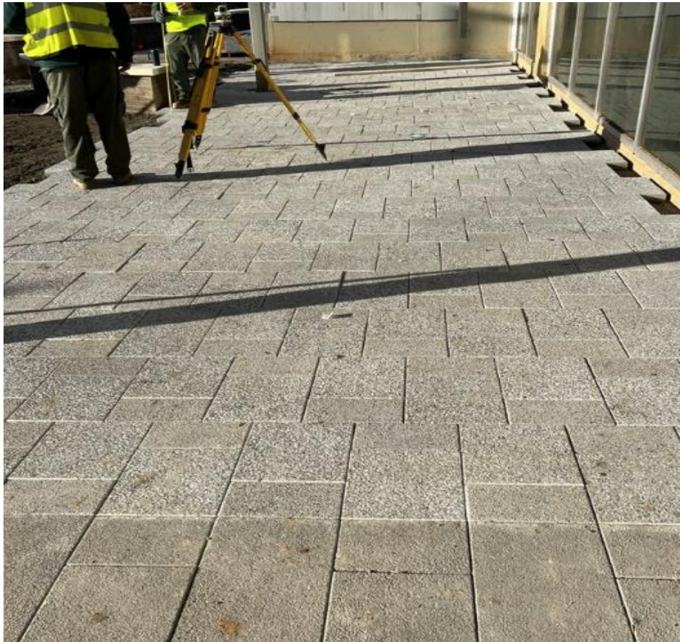
Pavers at Plaza
