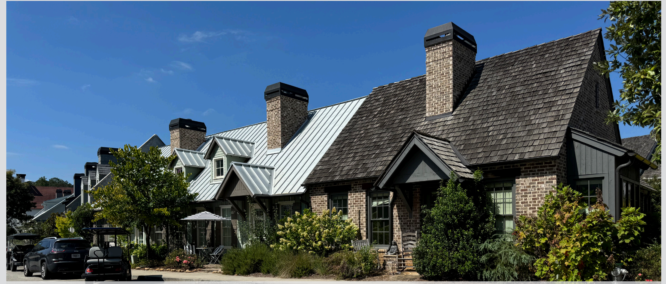
Townhomes with varying roof materials to differentiate units while remaining attached
