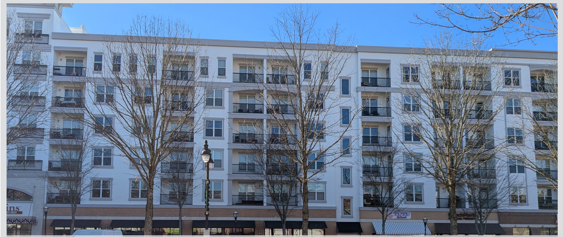
Traditional articulation and a very flat facade
