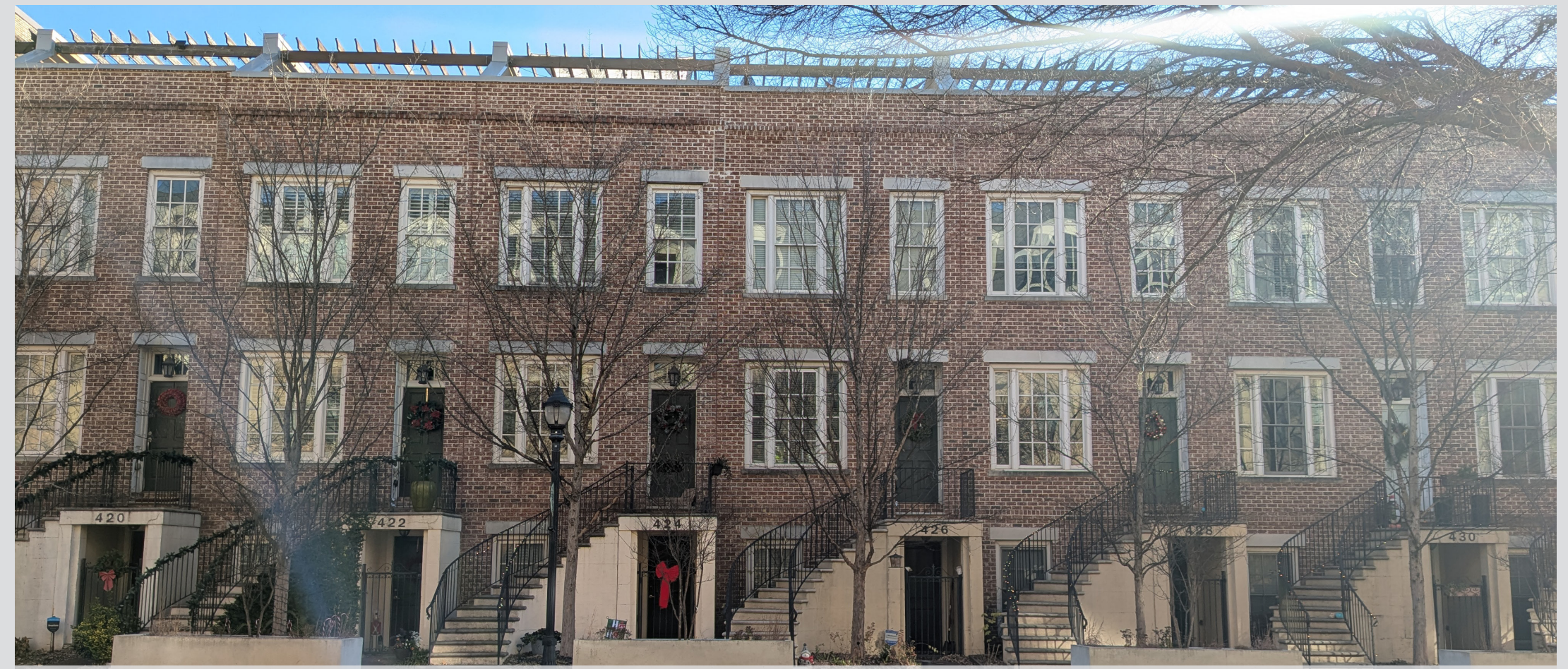
Townhomes constructed with a single material, appearing as one continuous building
