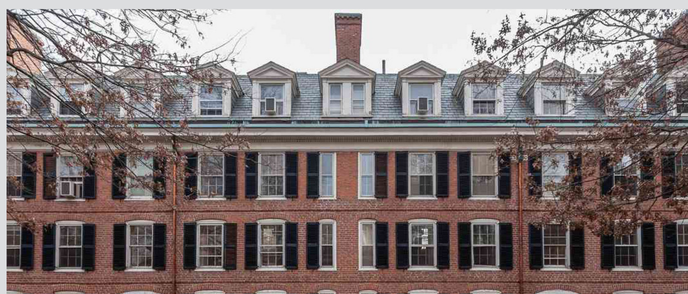
High transparency while maintaining a sense of enclosure with a heavy material
