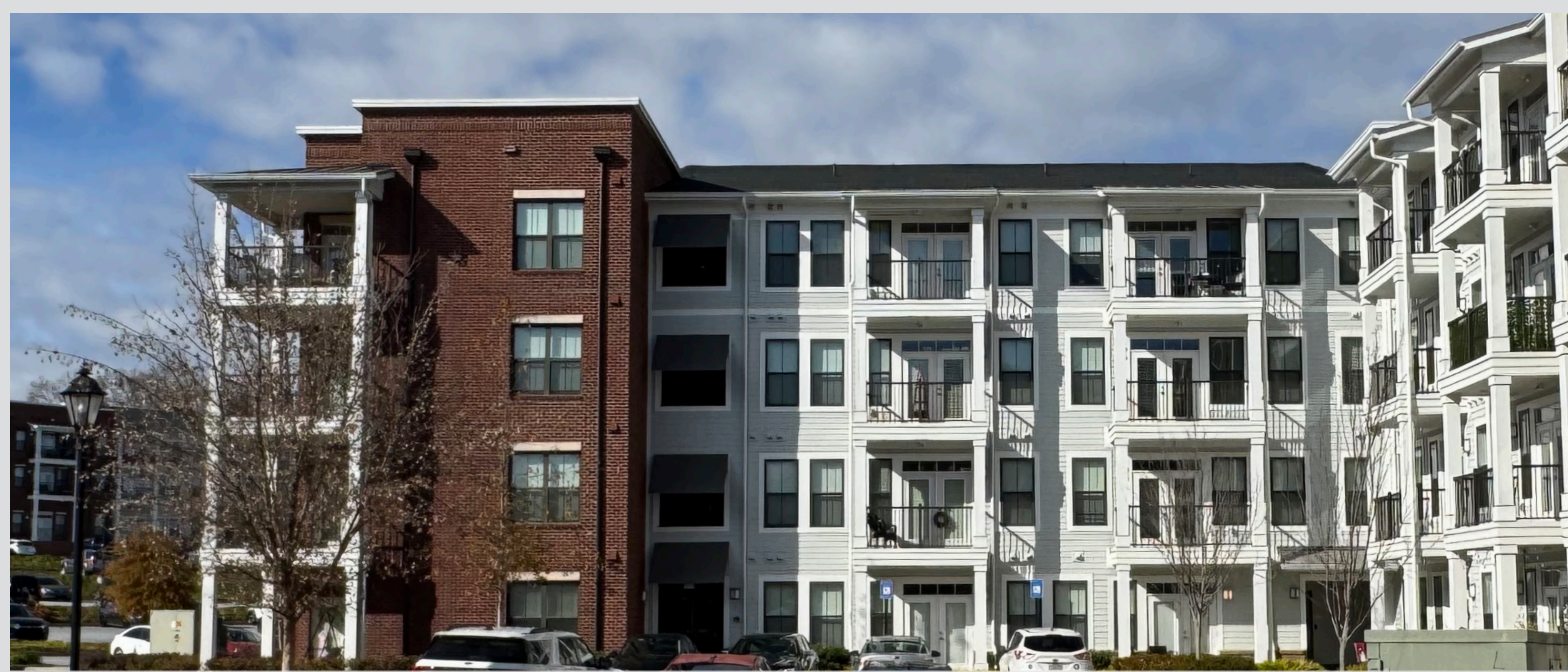
Articulation with protruding balconies and facade breaks at the corners
