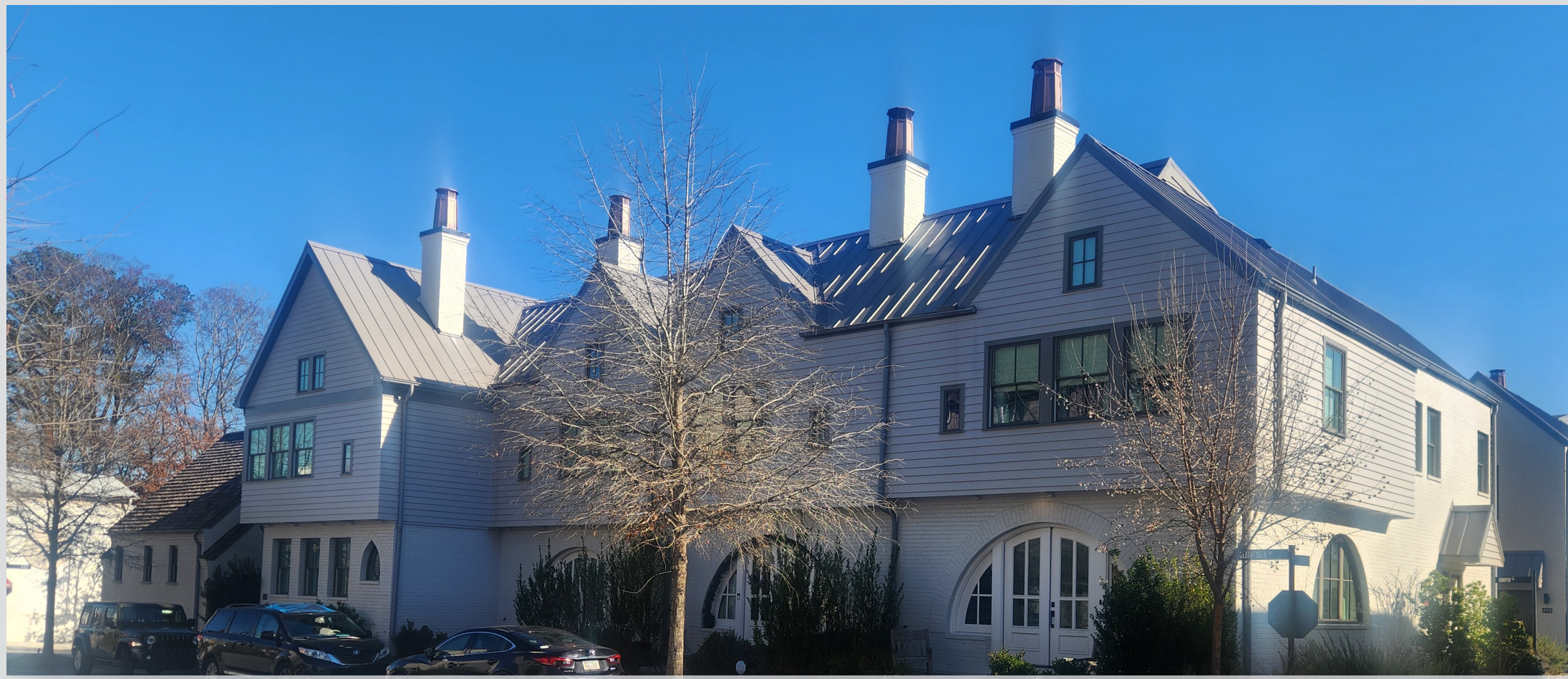
Townhomes arranged in a non-linear fashion, adding variety to the overall massing
