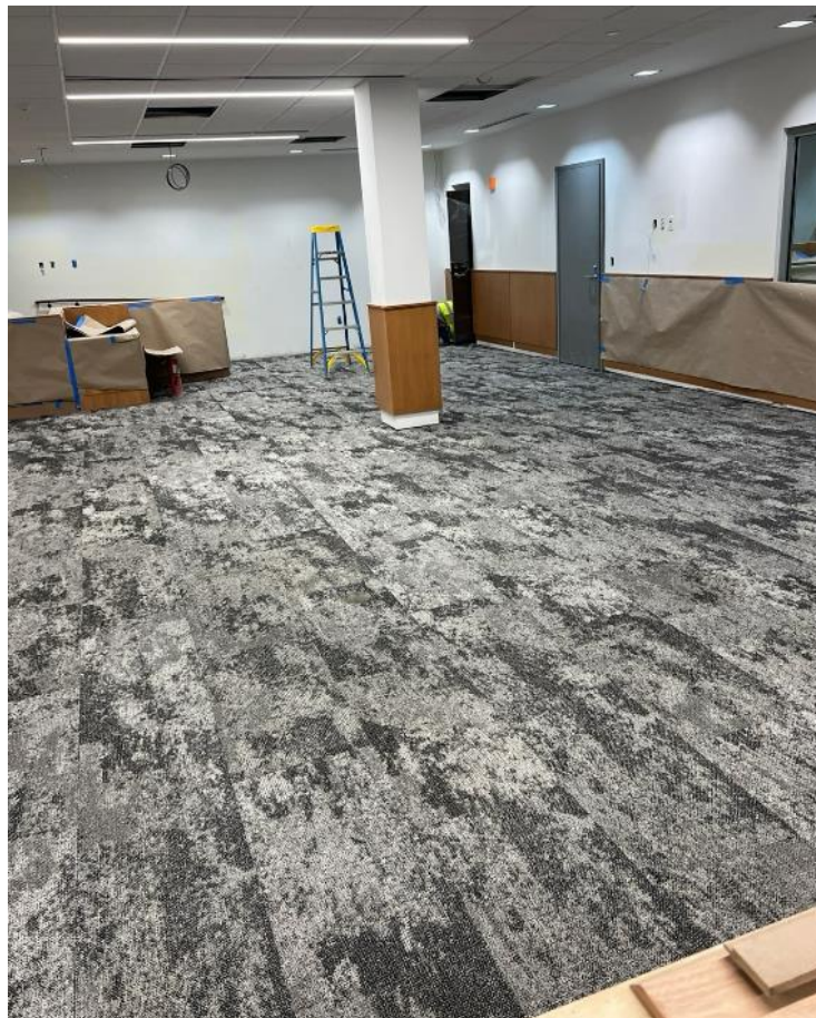
Finishes at Courtroom
