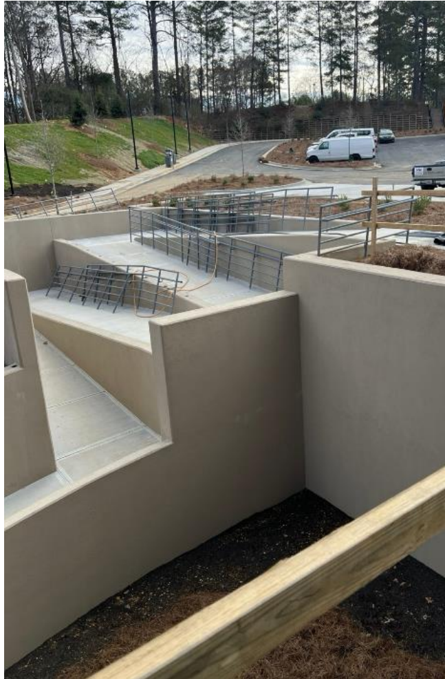
Railings at Ramps
