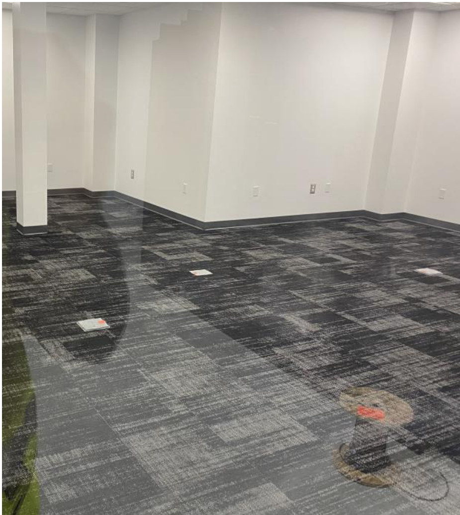
Flooring at IT
