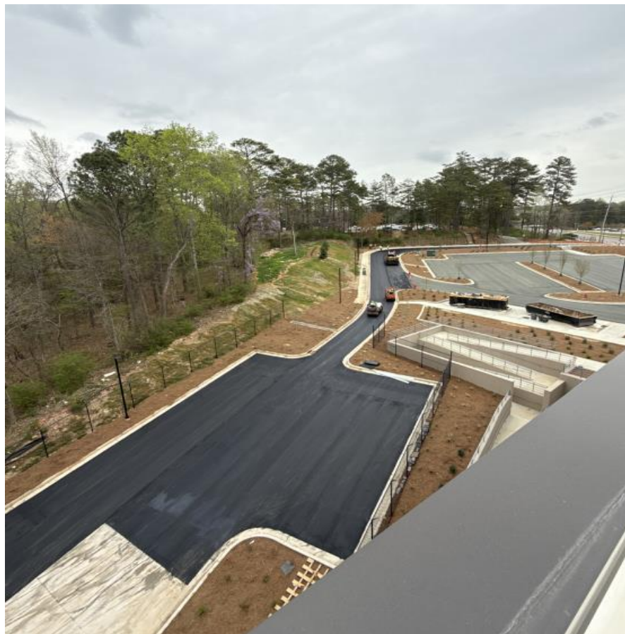
Asphalt Topcoat
