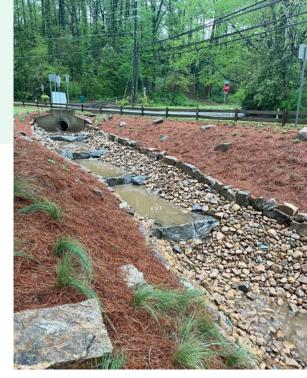
A contractor was selected to remedy the failing swale. The existing swale was dug deeper, adding twenty tons of river rock to help filter sediment and improve water flow. Twenty-eight tons of boulders were used along the sides of the swale to reduce the slope and slow the force of stormwater runoff.
