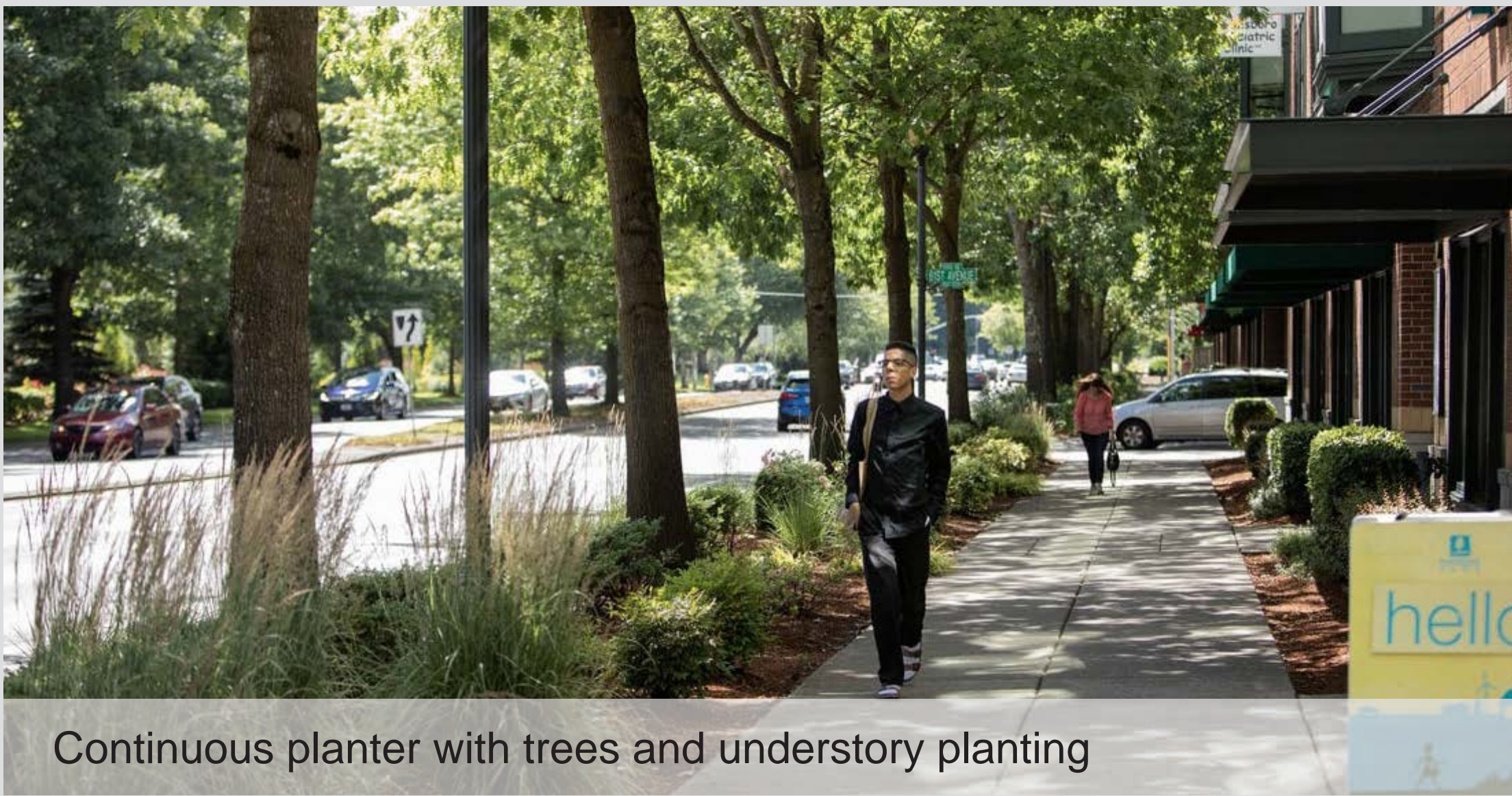
Streetside bioretention facility
