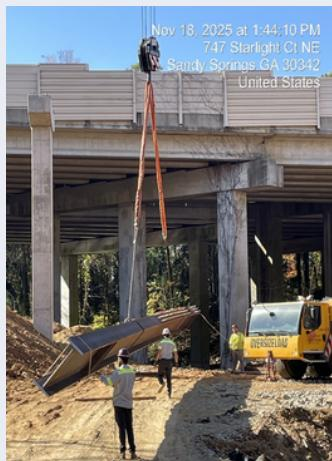
Construction on the PATH 400 multi-use path continues to move forward. In the photo on the right, you can see active wall construction taking shape as crews build out key structural elements. The photo on the left shows crew members setting beams at the southern end of the project, marking another important step toward completing the new trail connection.
