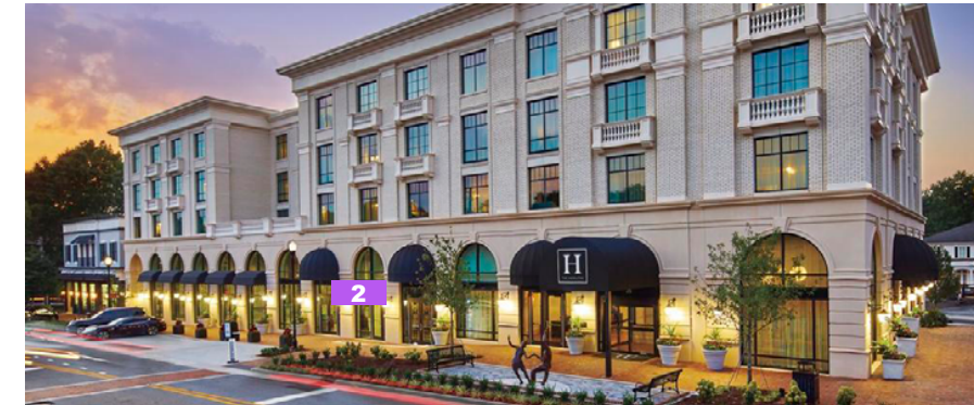
2 Use Arcades or Colonnades to provide shade and rhythm while maintaining continuity. (5.C.5-A2)
