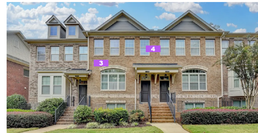
3 Use a consistent material palette (e.g., brick, wood, stucco) that reflects local character (5.C.5-A3)
