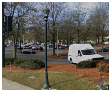
Cooper Generation ACN Post Top Fixture on Hapco 12' York Series Lighting Pole Color: "Dark Green" by Valmont Industries
