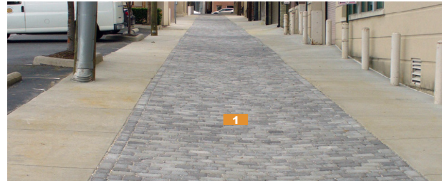
1 Permeable paving at center of alley captures stormwater (4.B.4.-C1)
