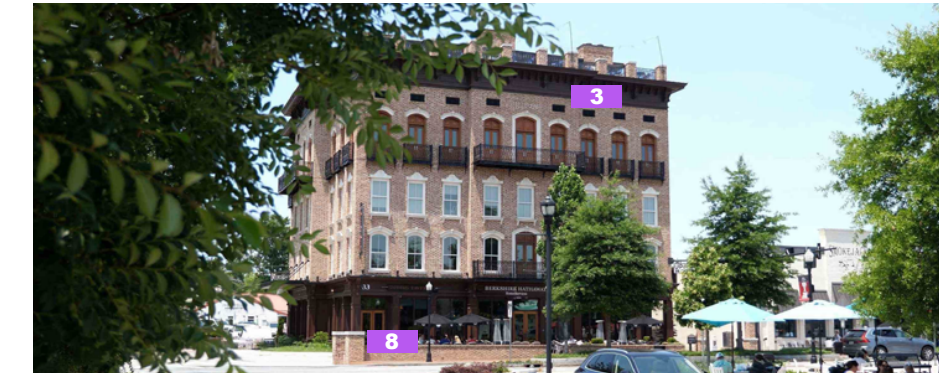
3 Use a consistent material palette (e.g., brick, wood, stucco) that reflects local character (5.C.5-A3)
