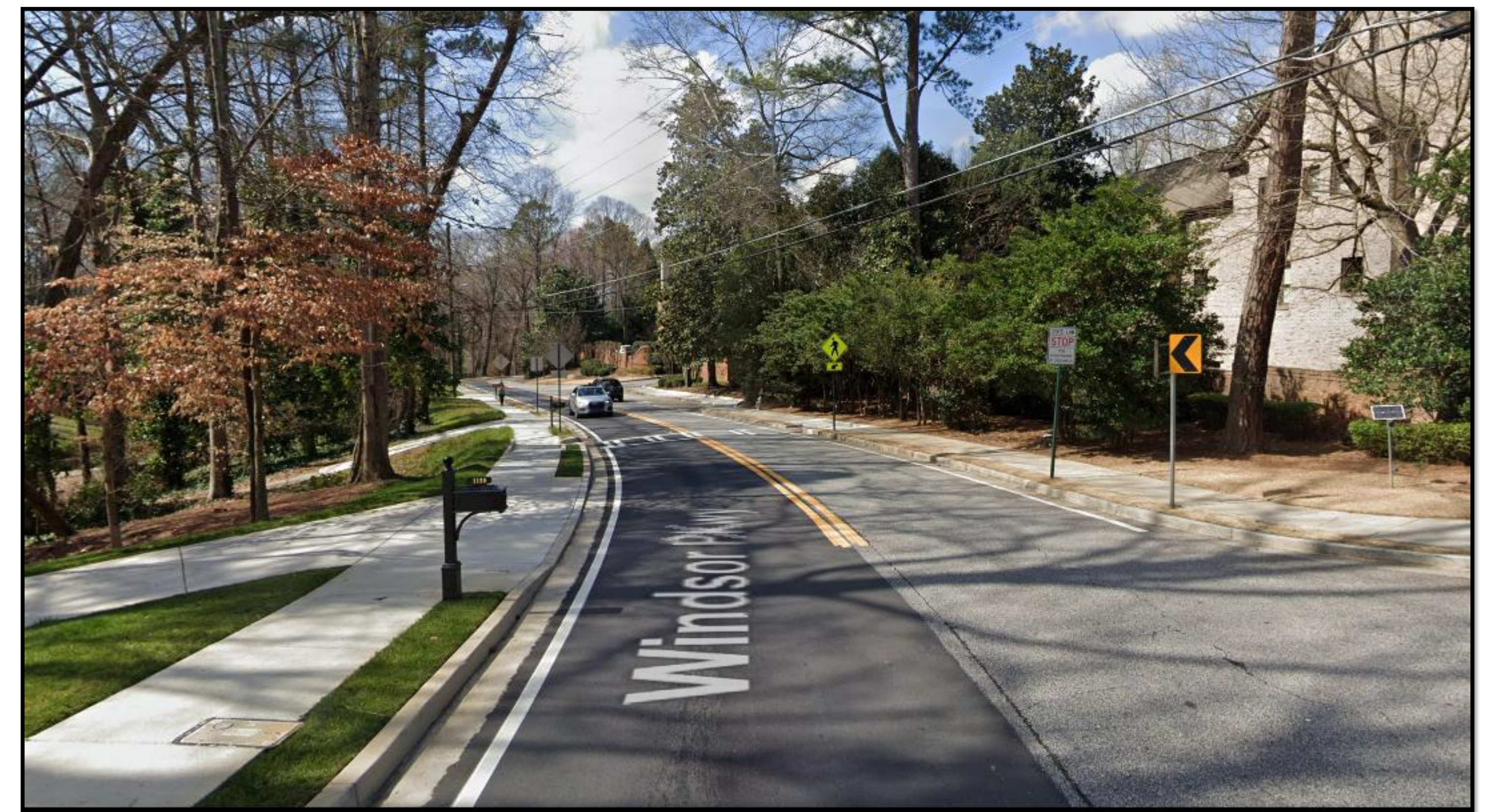
Before and after photos of sidewalk project on Windsor Parkway funded by TSPLOST 2016
